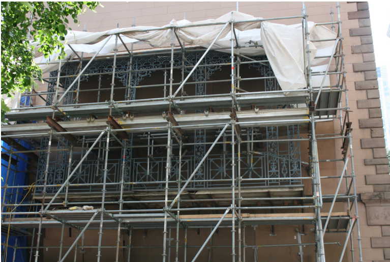
Scaffolding surrounding the East Balcony, July 2012.
